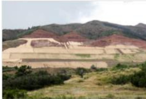
Work to reclaim the century-old Pikeview Quarry northwest of Colorado Springs is nearing completion
