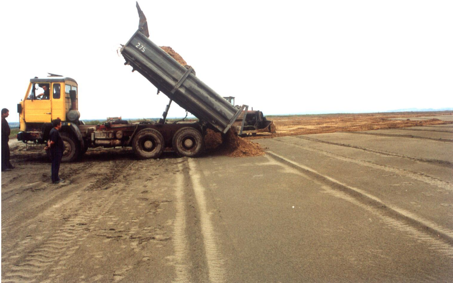
Introducing the mineral soil layer on hydrosilicate cover - technical phase of bigger scale method introduction - 2001 year, Zinc and Lead tilings pond, Bukowno, Southern Poland, photo by M. Pietrzykowski
