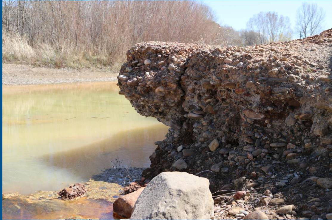
Ferrocement at the local swimming hole on Belt Creek
