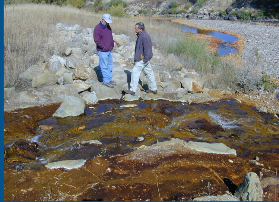
AMD Discharge to Belt Creek with heavy iron deposits
