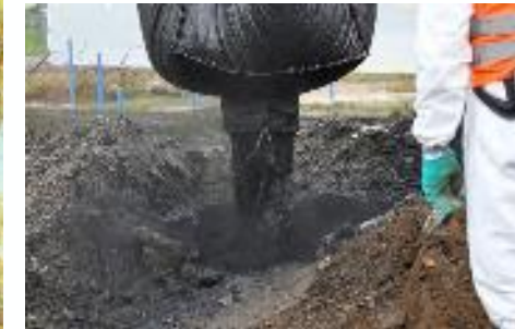
Apply MercLok™ to soil, sediments or mixed wastes
