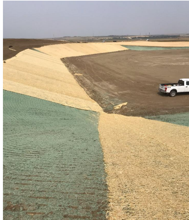
Grading + Soil Roughening + Hydroseeding + Matting
