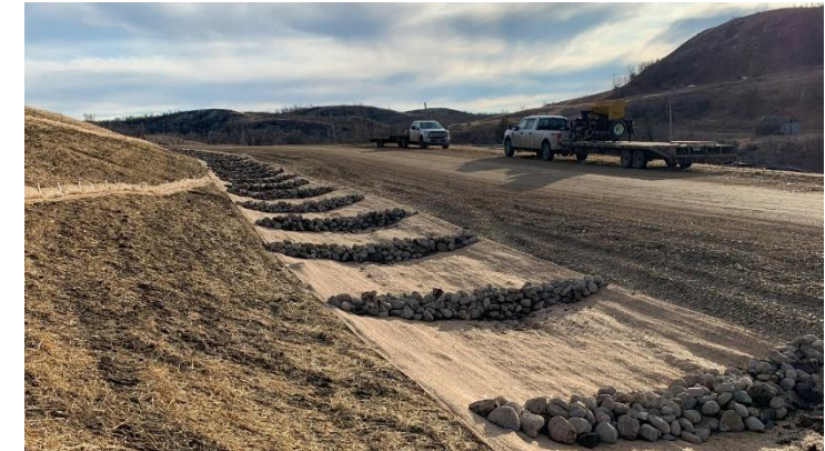
Channel + Matting + Riprap Check Dams Fiber Rolls + Straw Mulch
