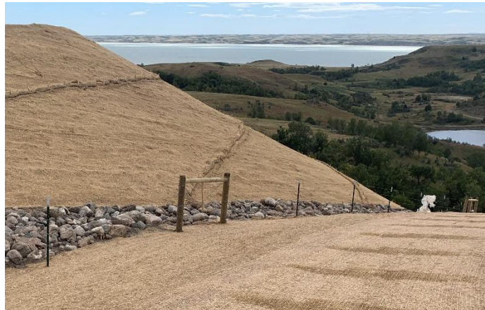
Channel + Riprap Fiber Rolls + Matting
