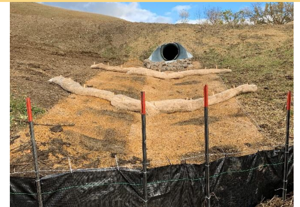
Riprap + Matting + Fiber Rolls + Silt Fencing
