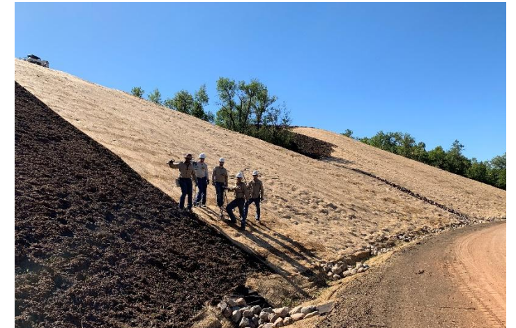
Grading + Compost Blanket + Matting
