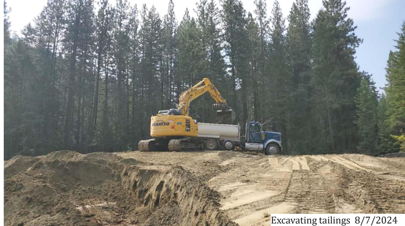
Removed tailings in contrast to adjacent forest 8/7/2024
