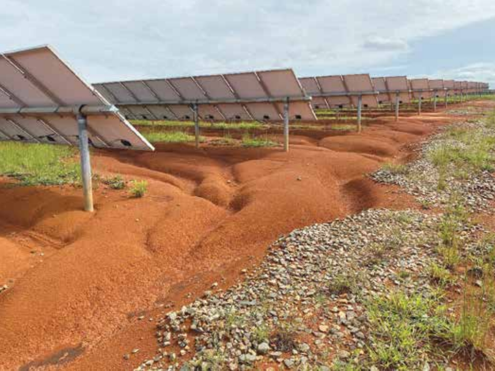
SWCA stabilized large-scale erosion at the Davidson County Solar Farm in North Carolina by armoring concentrated flow areas, redirecting runoff to prevent erosion, and implementing a native plant and pollinator re-vegetation strategy for site stability. Image shows project before stabilization for erosion.
