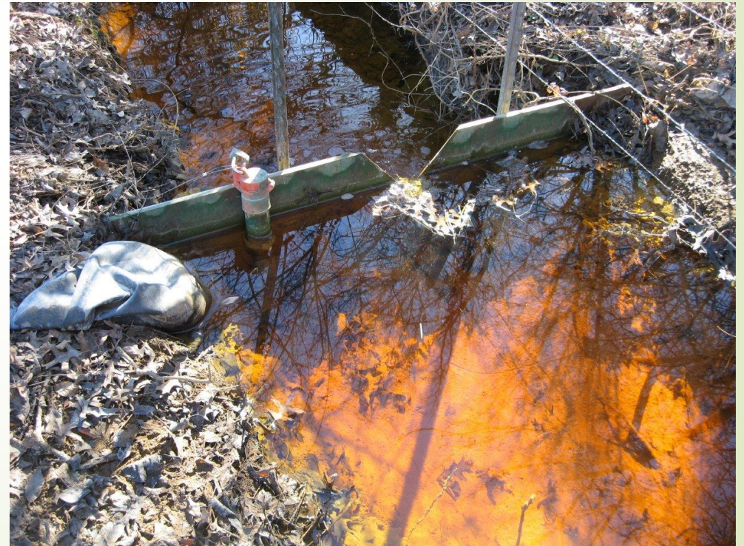
Wier installed at AMD site D-2
