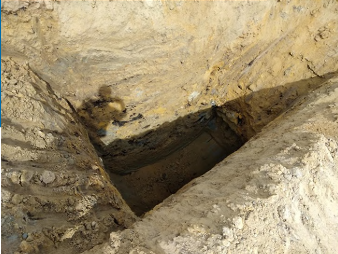
Test Pothole
