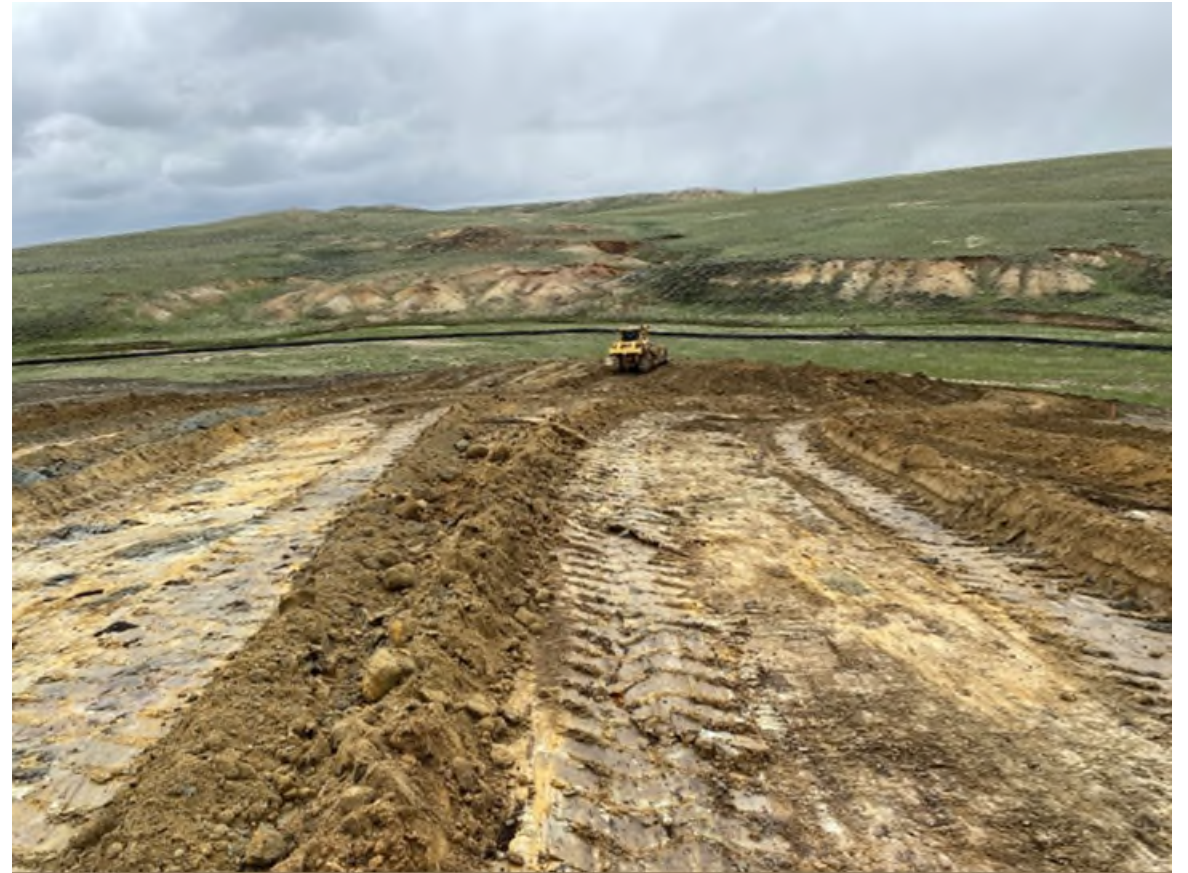
Subgrade Excavation
