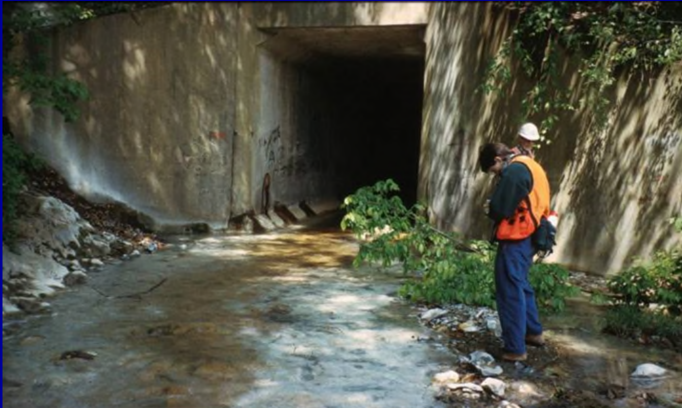
Culvert beneath I-64 in Clifton Forge
