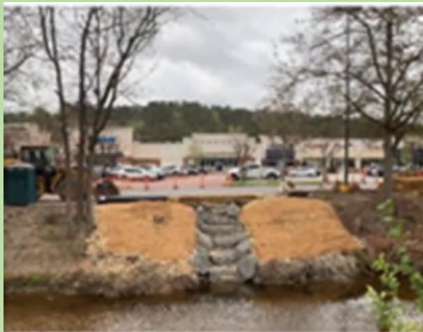
Installed and stabilized rock cascade
