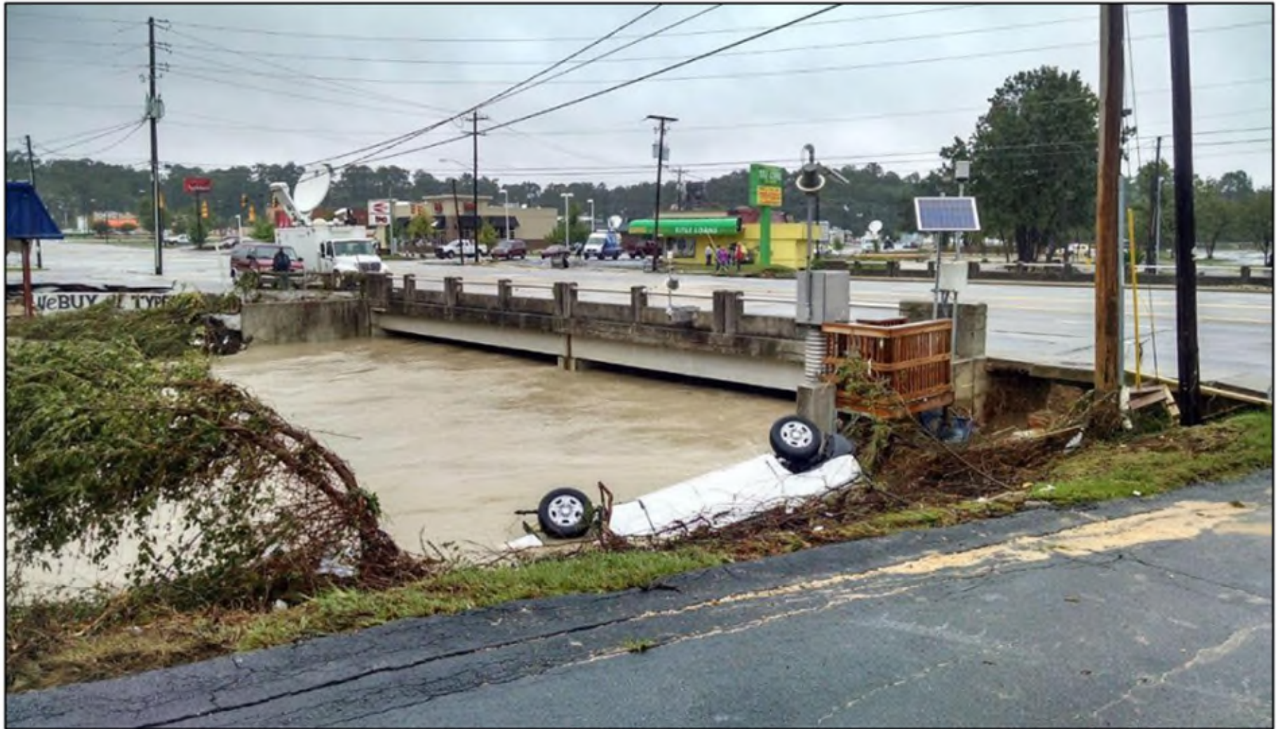
Figure 5: Conditions at U.S. Geological Survey streamgaging station 02169570, Gills Creek at Columbia, SC, on October 5, 2015. Source: USGS
