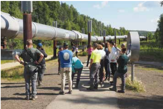
Figure 17. The Alyeska Pipeline viewing point. The Alaska Oil Pipeline is elevated for the most part and has cooling fins to prevent the permafrost from being impacted. The pipeline is the reason for essentially any infrastructure north of Fairbanks.
