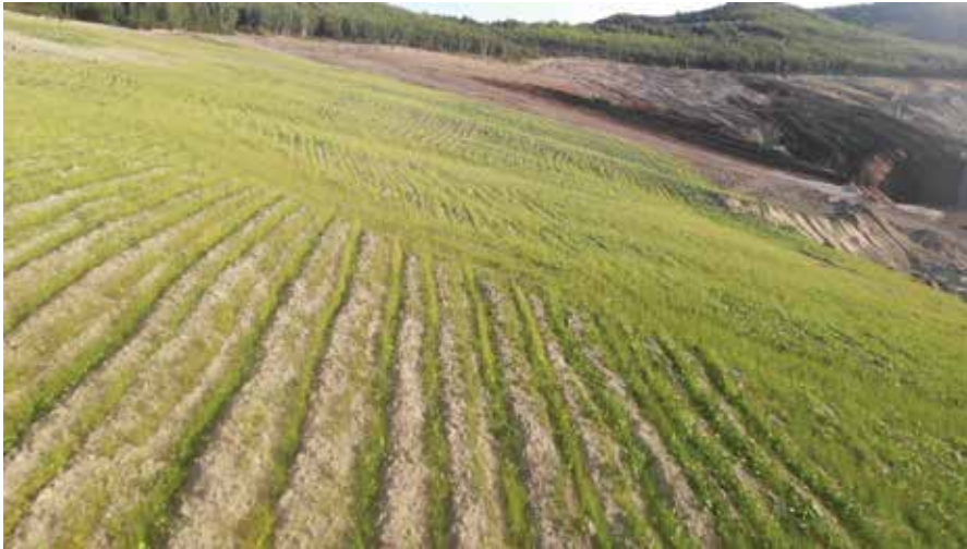
Figure 3. Furrowing and seeding at Two Bull Ridge in early June 2021 is shown in the foreground with active regrading in the background. Two Bull is across the valley from Poker.
