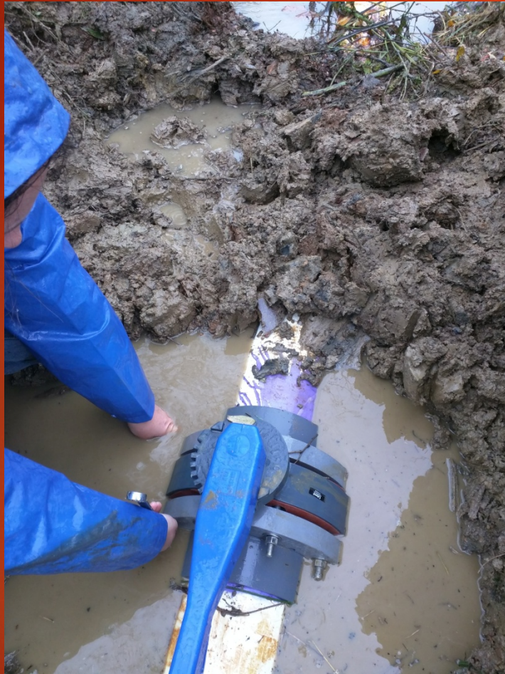
Settling pond 8" bypass valve replacement and removal of E&S controls left in place from initial system construction
