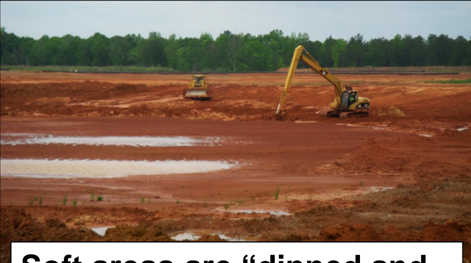
Soft areas are “dipped and spread”, and dozers spread the slimes to aid in drying.
