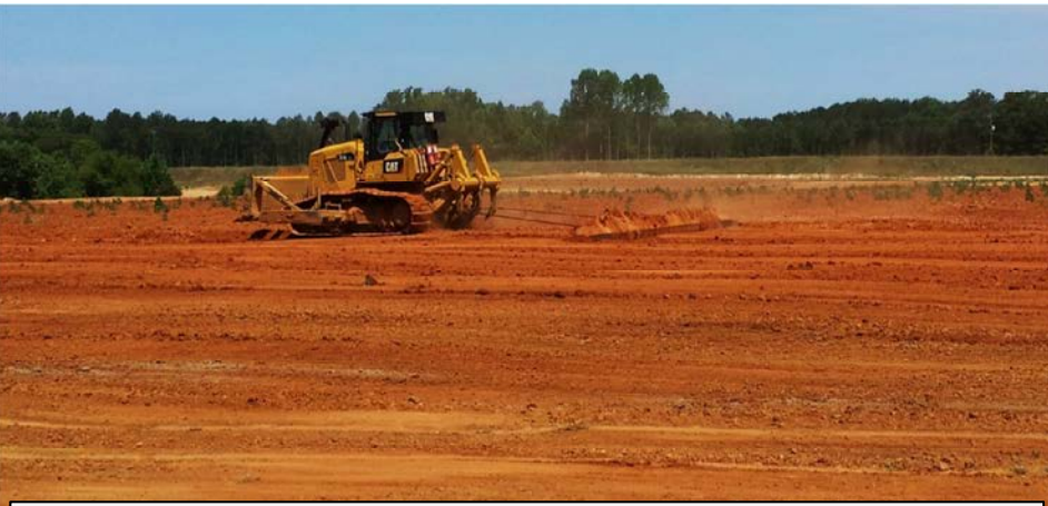
Land leveled with steel beam
