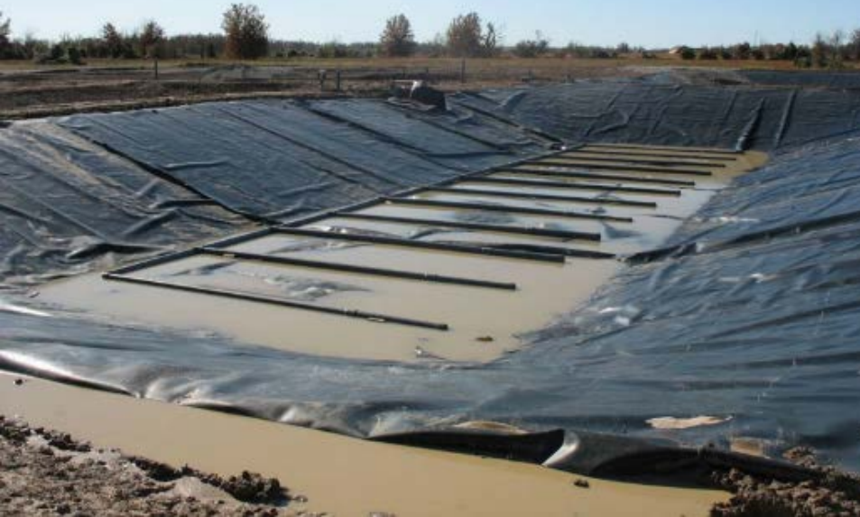
MRPTS vertical flow bioreactor, under construction, fall 2008
