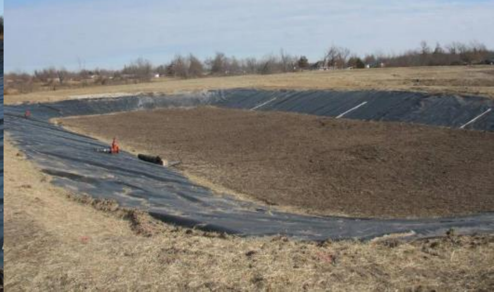
MRPTS vertical flow bioreactor, before flooding, fall 2008
