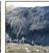
2 - Erosion along a coal culm pile approximately 51 feet high, immediately adjacent to Good Spring Creek
