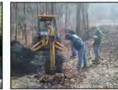
4 - Top trench dug in existing floodplain. All material excavated from the trench was fine coal material; no native soils or historic floodplain soils were found in the trench
