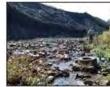
1 - Erosion along a coal culm pile approximately 51 feet high, immediately adjacent to Good Spring Creek
