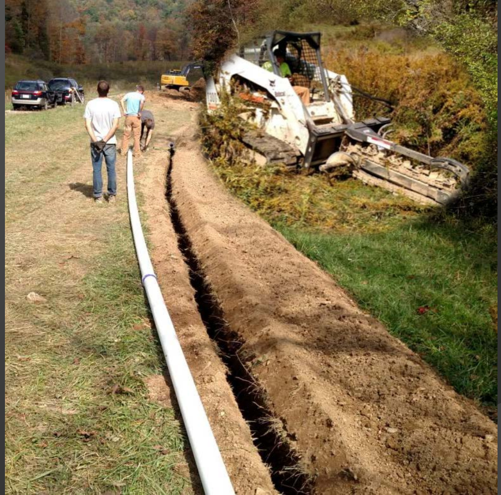
1,300' 4" Air line with positive drainage
