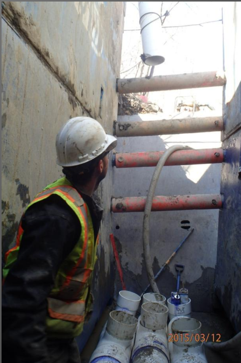
Vertical pipes between shoring
