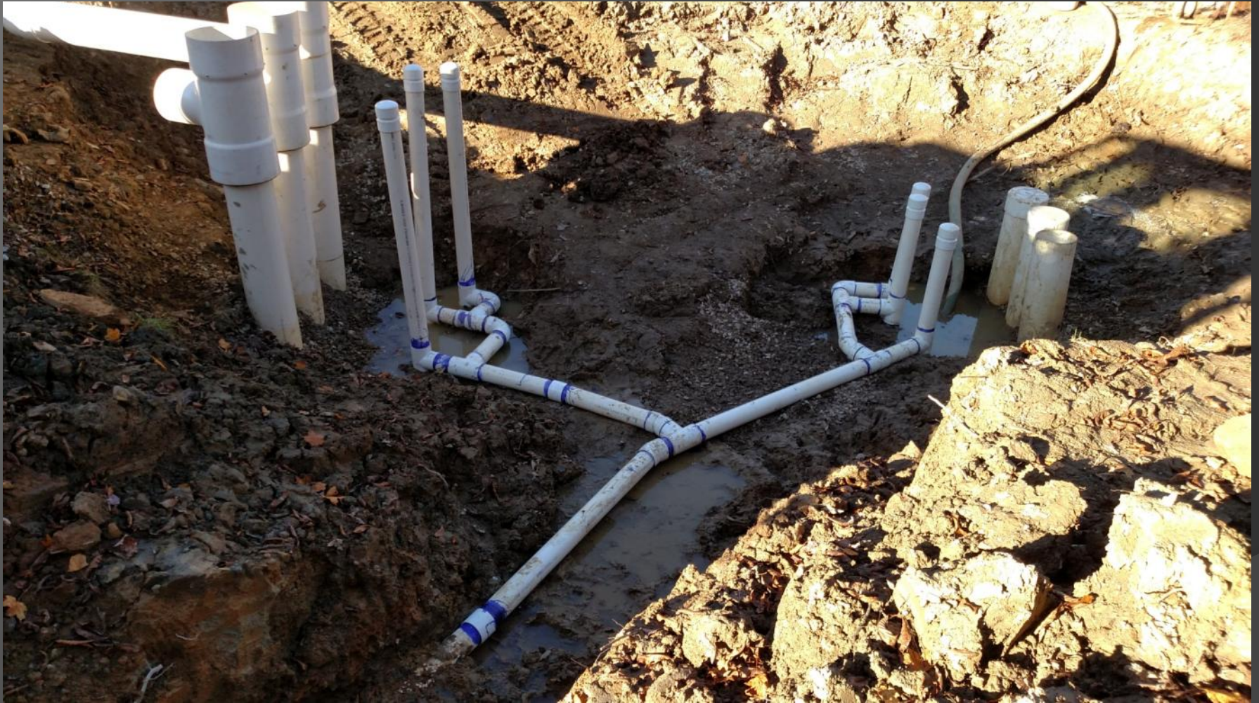
Air line manifold
