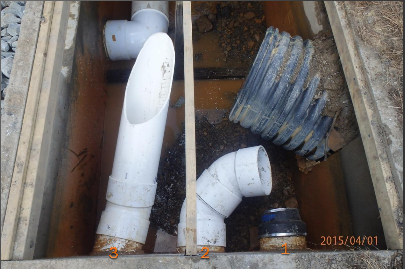
Inlet control for variable-flow sequential operation
