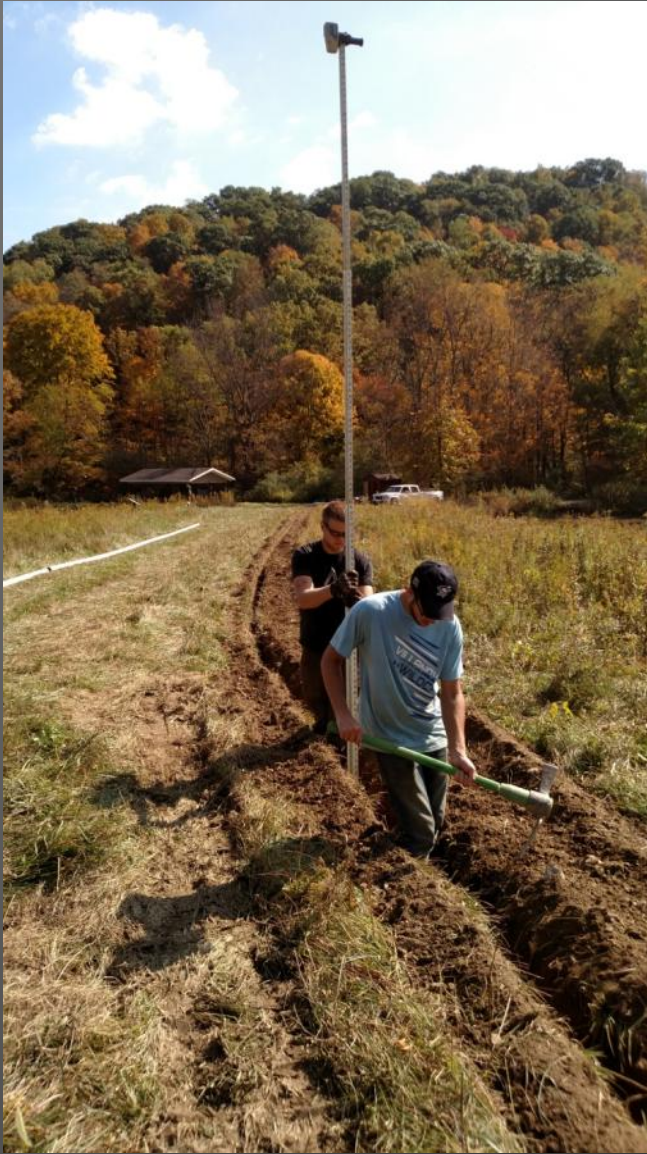
1,300' 4" Air line with positive drainage
