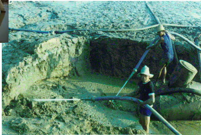
Reclaiming by hydraulic dredge pump, ----- Popular reclamation technique
