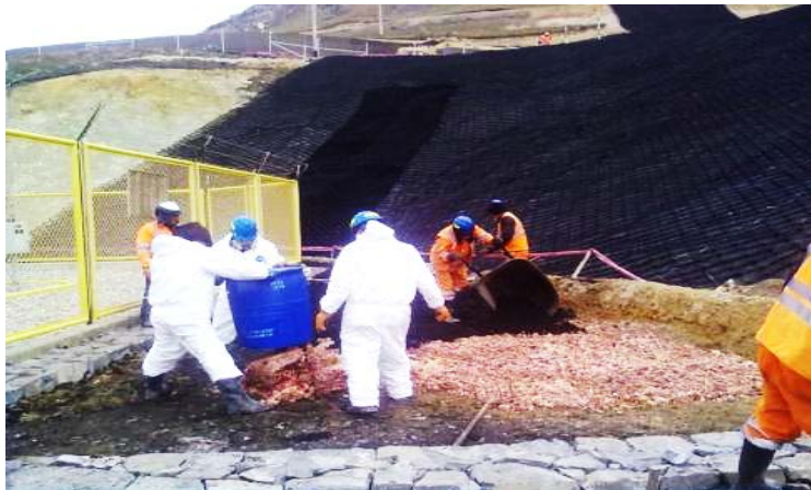
3) Incorporation in revegetation process
