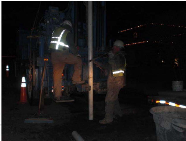
4 inch PVC casing installation
