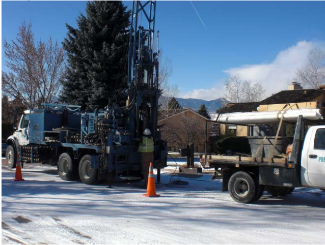
CSM 75 drill rig setup
