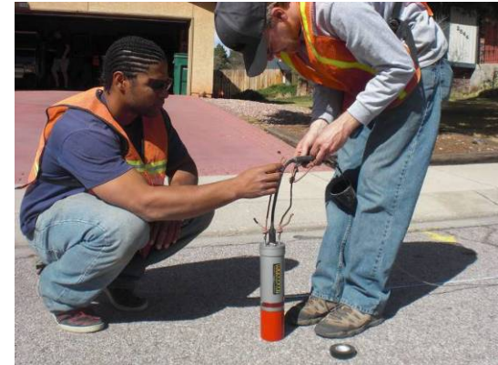
Sonar – Void scanning
