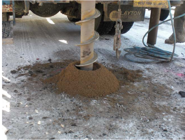
Drilling through ~ 40 ft sand
