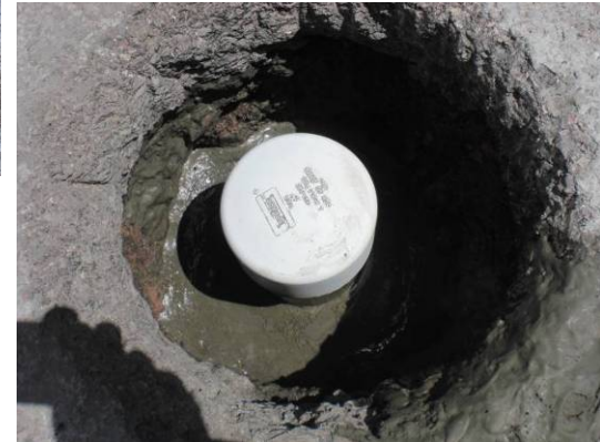
Casing/grout setup w/ 10% bentonite
