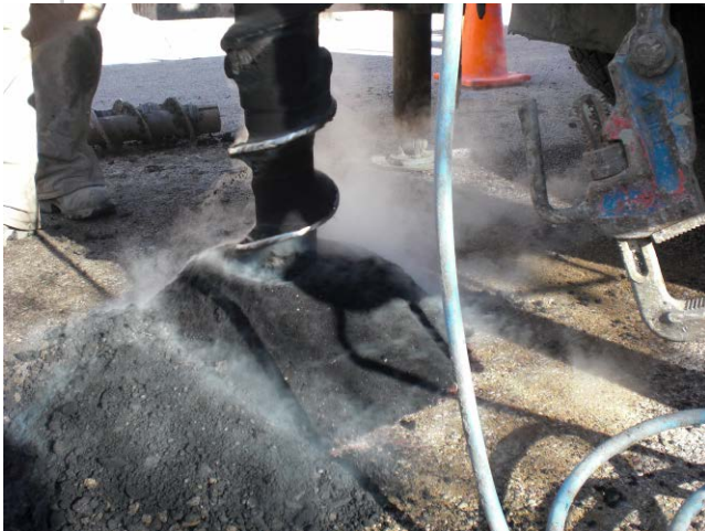
Drilling through ~ 7 ft coal
