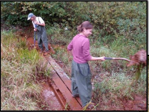
Successful vegetation led to overgrown level spreaders increasing channelization and adding to the problem rather than preventing
