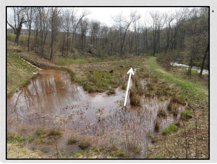
Channels within the wetland caused short circuiting = increased Fe in effluent
