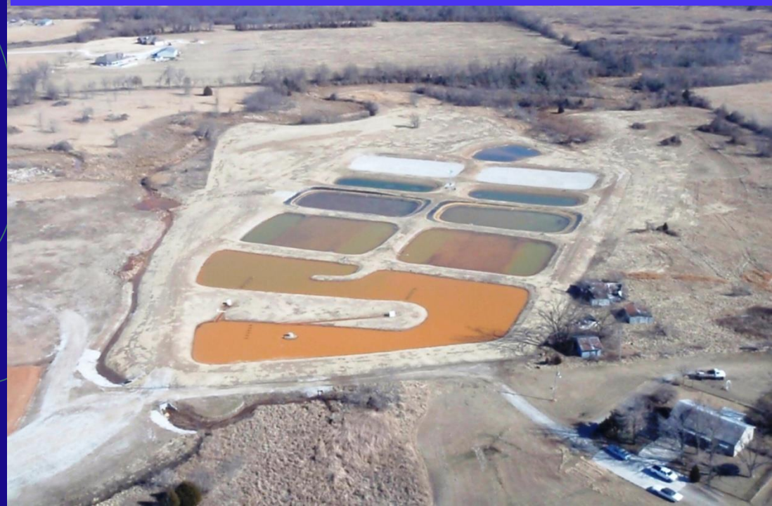
Mayer Ranch Passive Treatment System
