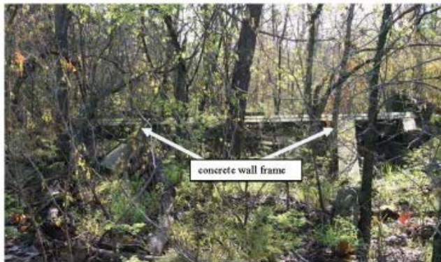
Figure A-9: St. Mary's of the Quapaw school, Building 2 (1915 Dormitory Building), view east of interior wall frame fallen into the interior of the structure.
