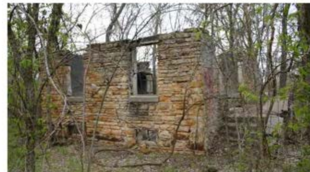
Figure A-19: St. Mary's of the Quapaw school, Building 8, view southwest of the east elevation and part of the north façade.
