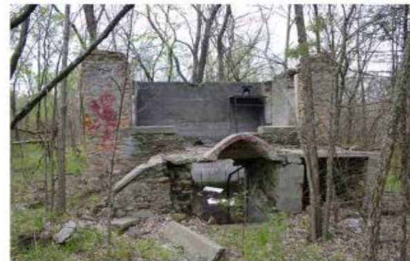
Figure A-18: St. Mary's of the Quapaw school, Building 8, view south of north façade with upper stairway landing with arched entrance of stairway to lower story. Alcove at right may have been for firewood.
