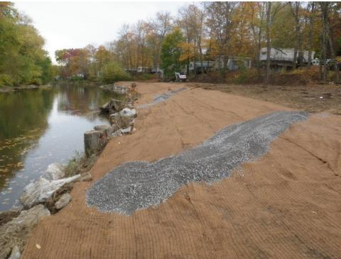
Coconut fiber erosion control blankets were laid along the bank and stapled in place to provide temporary erosion control until vegetation can take hold. Gravel was then placed on the designated paths to allow unrestricted access to the stream for fisherman and other recreational activities.
