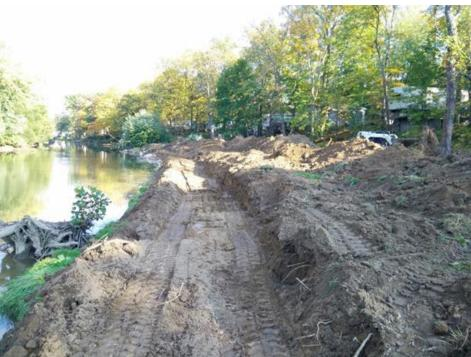
Photo to the left shows the initial phase of pulling back the embankment to allow for placement of rip rap and increase stabilization. Photo to the right shows a temporary bench used to transport and place rip rap along the toe of the streambank.
