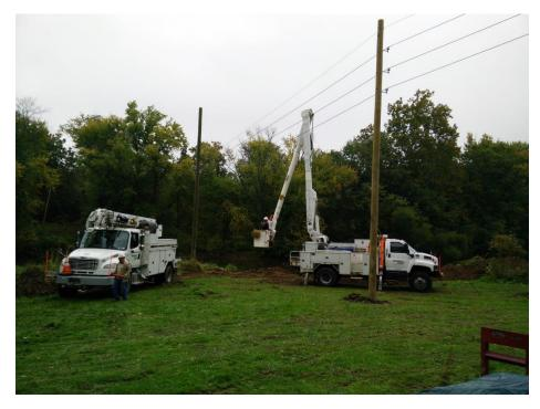
Photo to the right: Before the bulk of the construction could begin a power line had to be moved back from the stream bank. The photo to the left shows slumping that occurred due to the large amount of undercutting from the stream.
