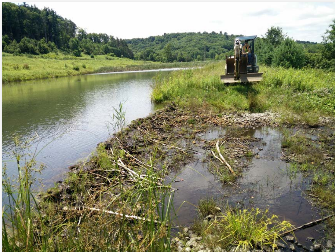
Beaver dam located at emergency spillway
