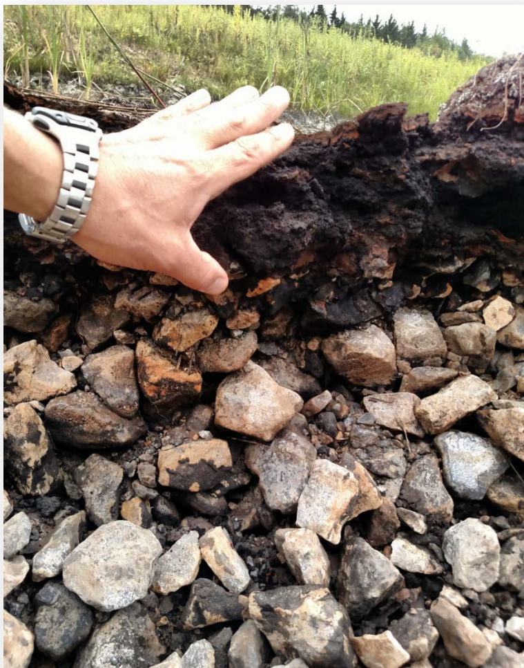
Sludge/stone layering prior to cleaning
