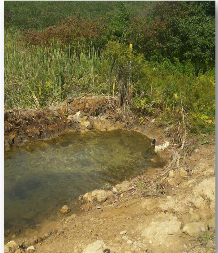
System outlet cleared of vegetation and outlet pool constructed.
