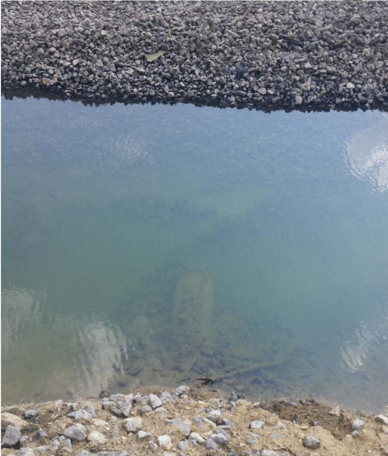
HFLB underdrain manifold replaced by outlet pool
