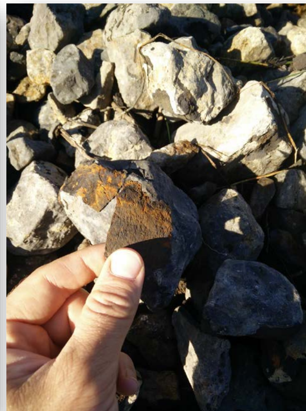
Fe & Mn 'flakes' on spillway limestone
