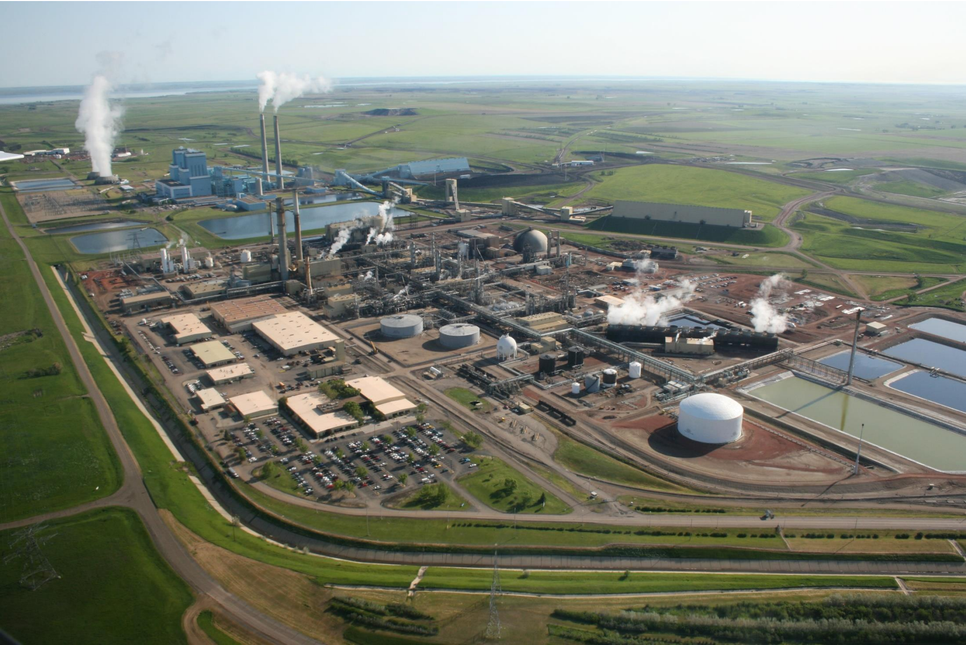
The Freedom Mine supplies fuel for Basin Electric Power Cooperative's Antelope Valley Station & Leland Olds Station, and feedstock for the Great Plains Coal Gasification Plant.
