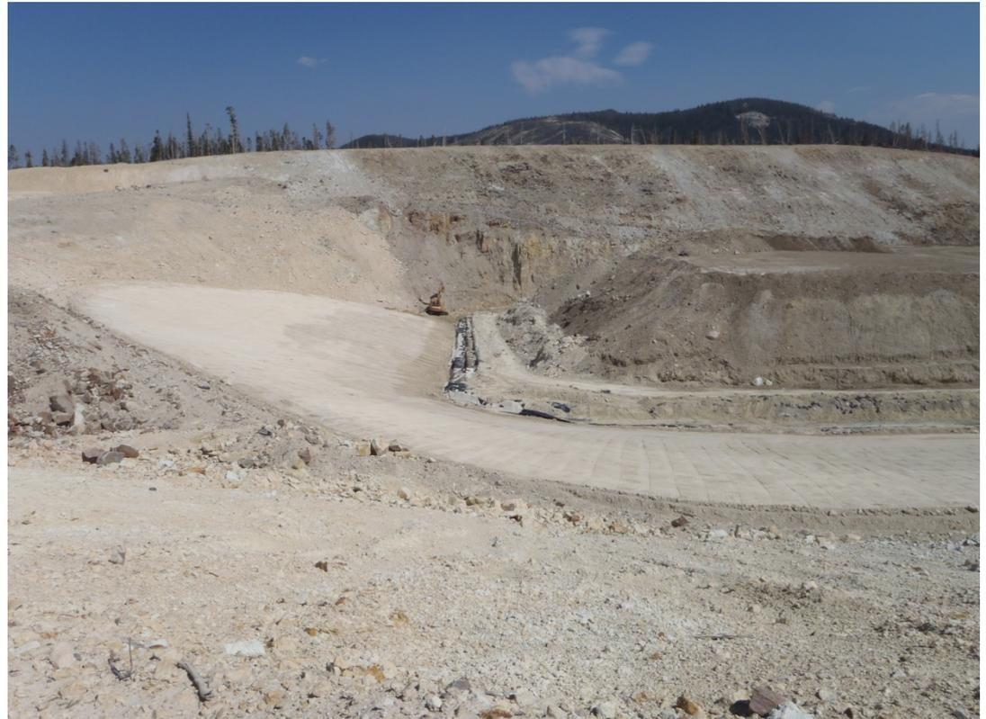
Final base grading of Cell 5 expansion to north and west
