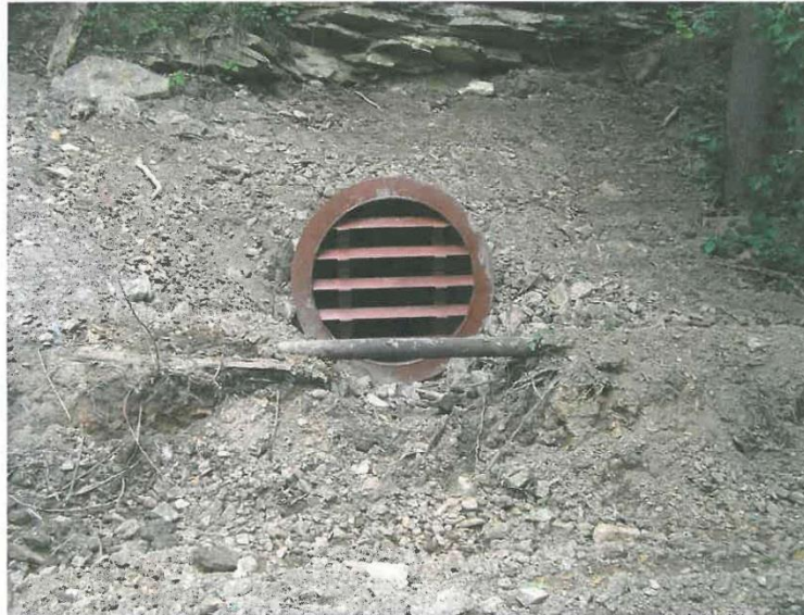
Postconstruction portals along access road
