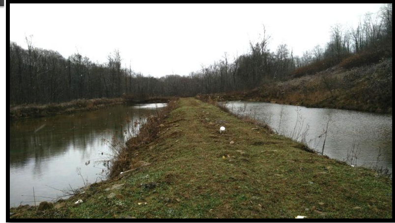
At Laurel Run #1 Vertical flow ponds (Top) and flush ponds (Bottom) were rehabilitated by Biomost, Inc. alongside the addition of a new VFP by Amerikohl Mining, Inc.
