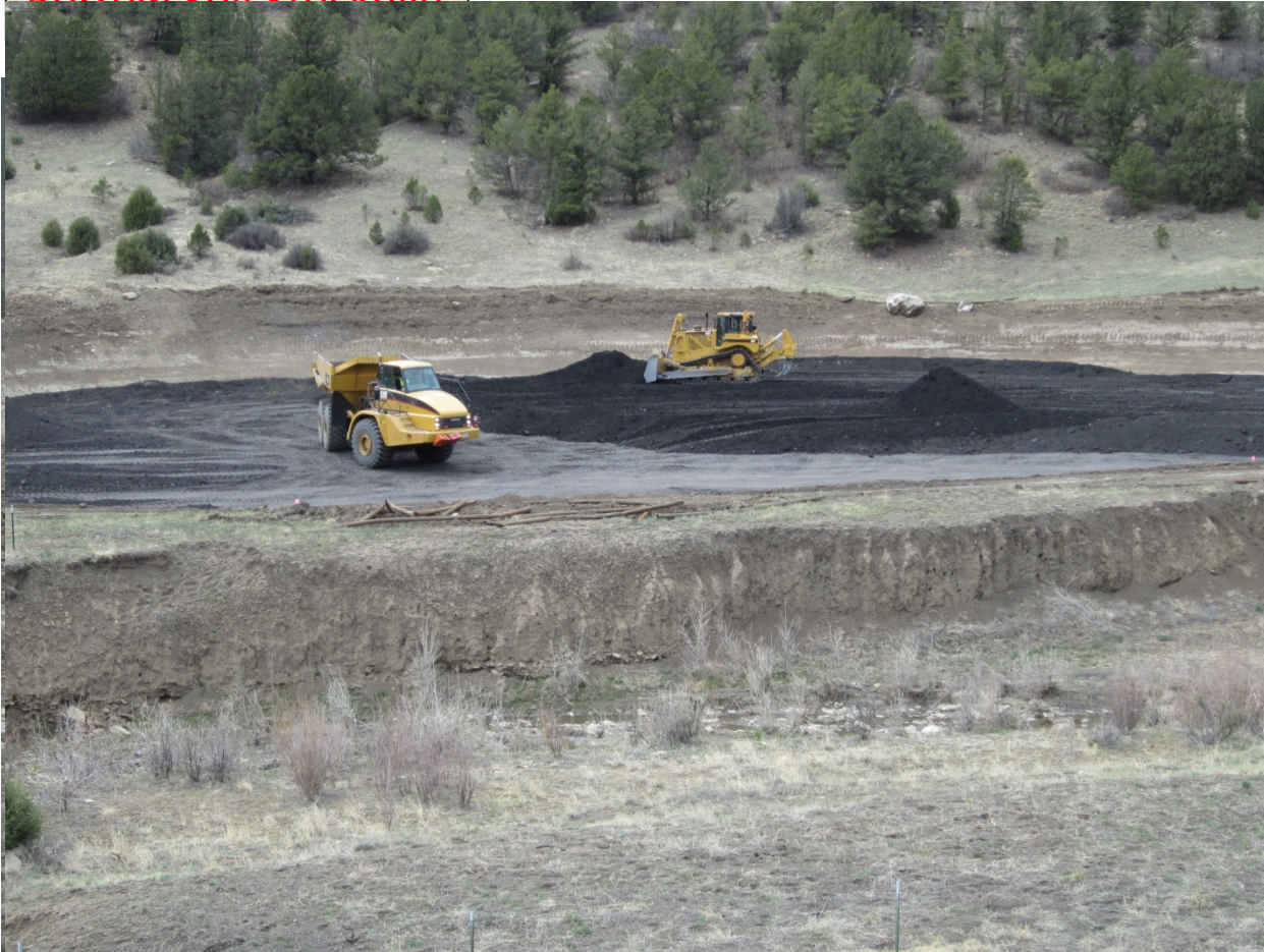
Borrow Soil Stockpile
