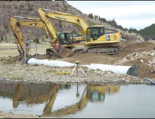
Setting Stormwater Relief Culvert
