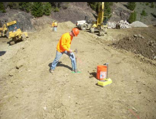
Compacted Earthen Core
