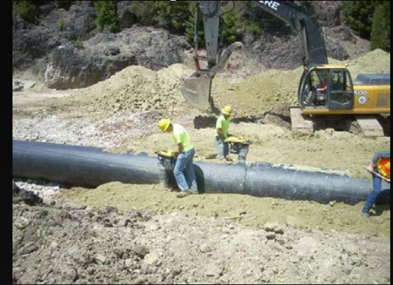
Compacting around Culverts
