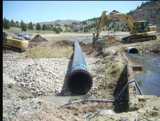
Setting HDPE Diversion Pipe
