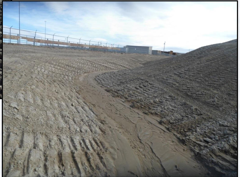
Channel Constructed in Cut
