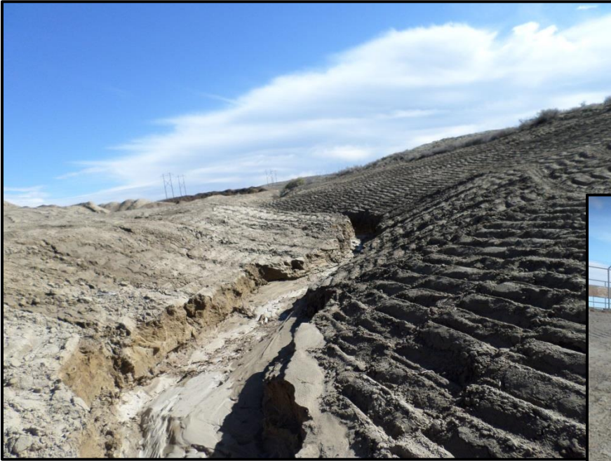
Channel Constructed in Fill
