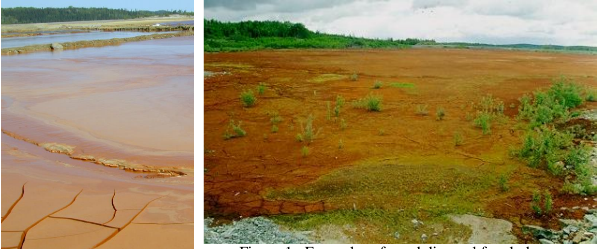
Figure 1: Examples of pond disposal for sludge.
