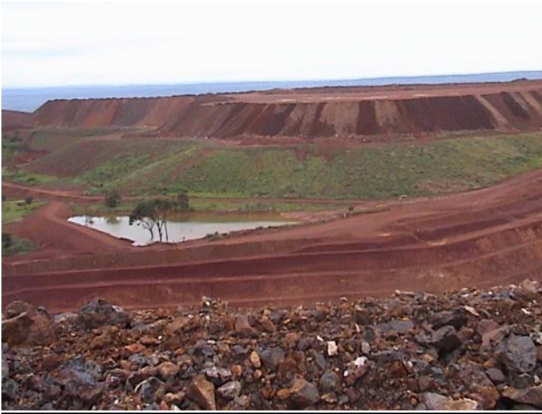
Figure 8: Ongoing contoured rehabilitation on Waste dump 8 at Kukuluma pit.
