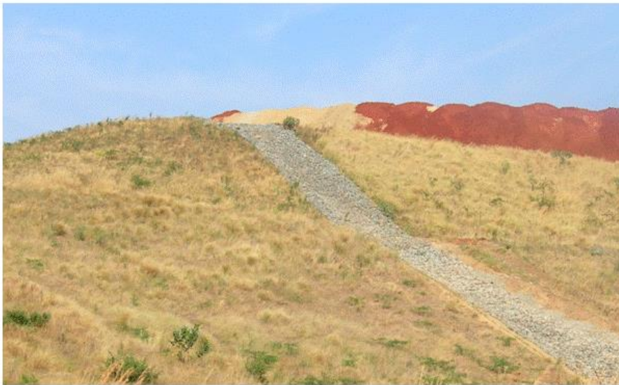
Figure 5: Nyankanga Waste dump showing one of the drainage channels that drain water off the dump slope
