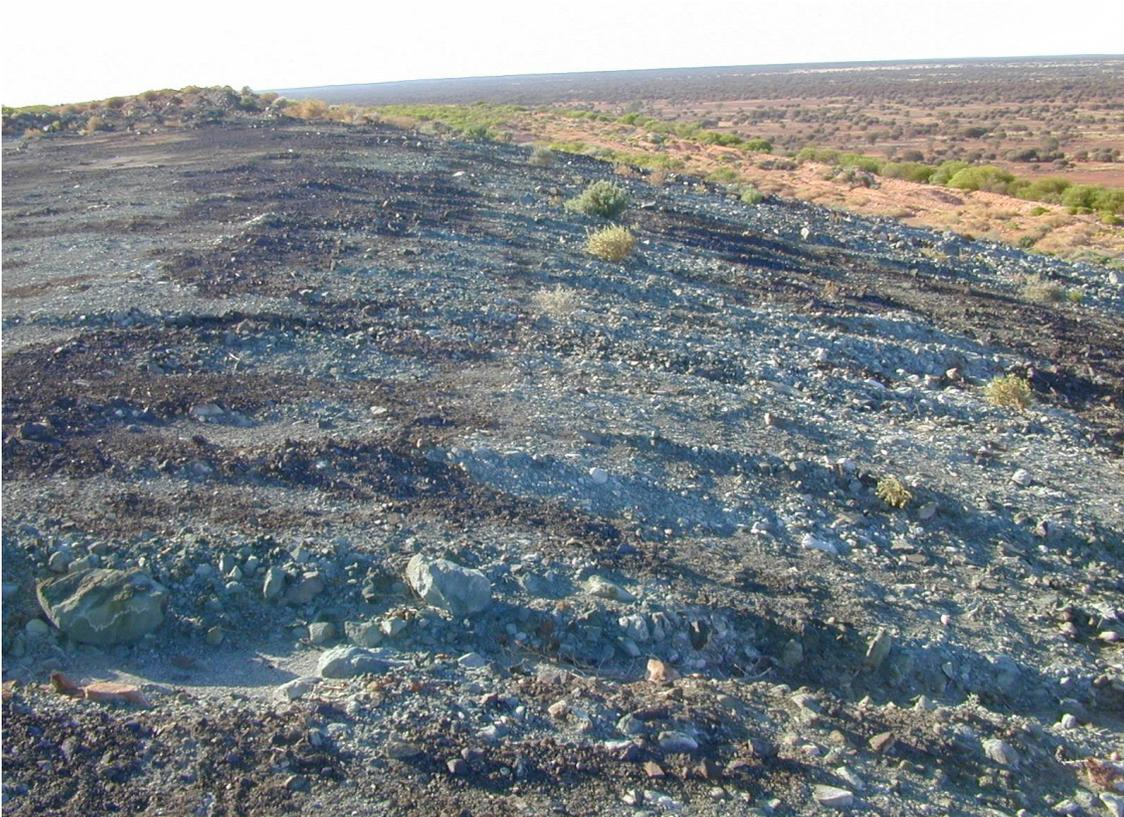
Figure 6. 'Black' staining on surface of dump face consisting predominantly of siderite/hematite precipitates.
