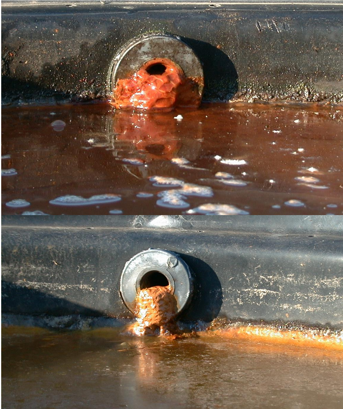
Figure 5. Photographs of the tank influent orifice showing iron oxyhydroxide crust precipitated at pH ~2.4. These low pH iron oxyhydroxides crusts may have played a significant role in the sorption and retention of arsenic from the influent ARD.
