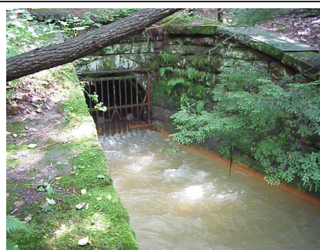
Figure 5d. Drainage from the Jeddo Tunnel mine discharge near Hazleton, PA. Flow at the tunnel is 3,100 l/sec (50,000 gpm) making it virtually impossible to detect any impact from a small remining operation.
