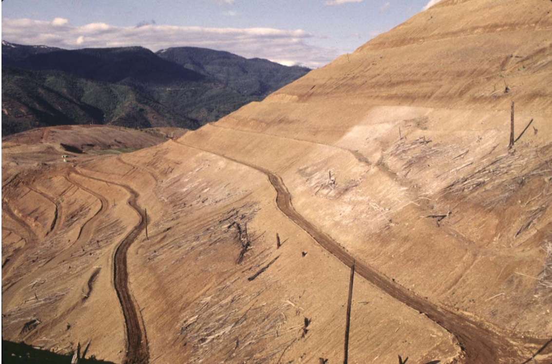
Figure 1. Pre-treatment hillsides environment in Government Gulch. Note construction of terrace benches spaced approximately 30 m apart. Steep slopes, exceeding 30 degrees (58 percent) and extending to over 500 meters in many places, dominate the site. Combined with extensive soil erosion, acidic reaction, and even steeper cut and fill slopes, the hillsides landscape is a difficult restoration challenge (photo taken in 1997).
