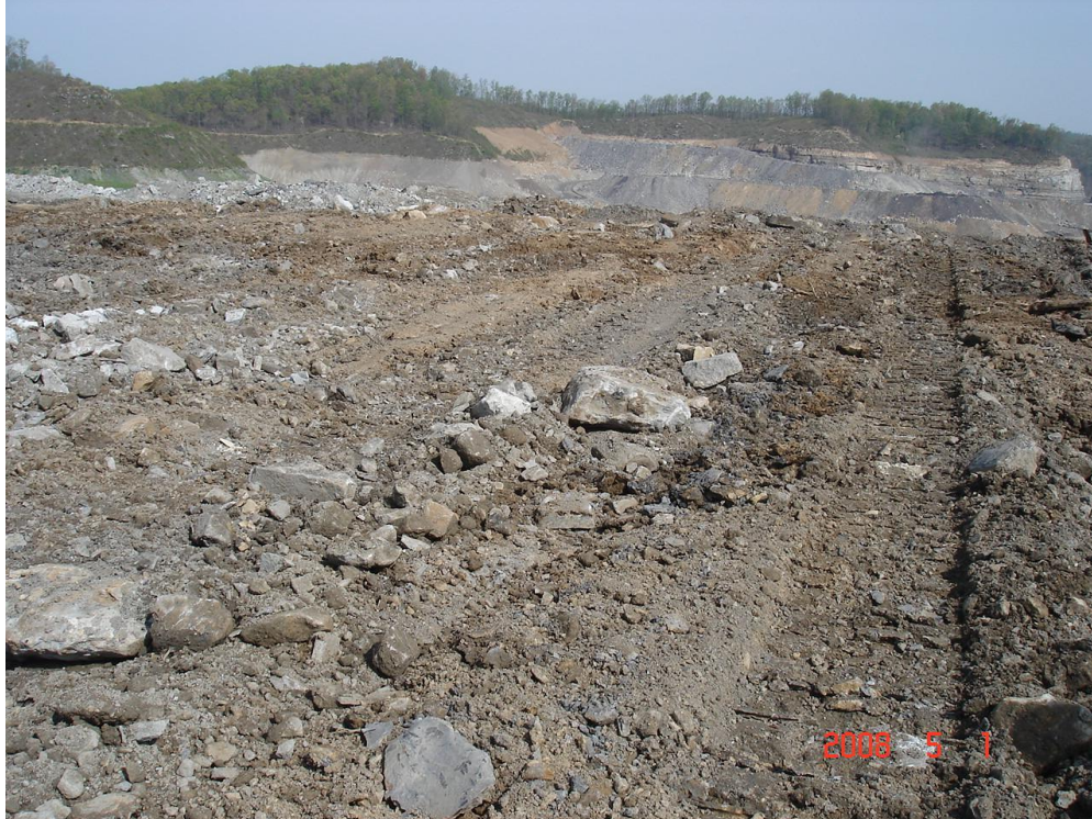
Figure 1. The 1-ha experimental area was constructed with primarily brown sandstone substrate, end-dumped with trucks, and the piles were flattened by one or two passes of a bulldozer.
