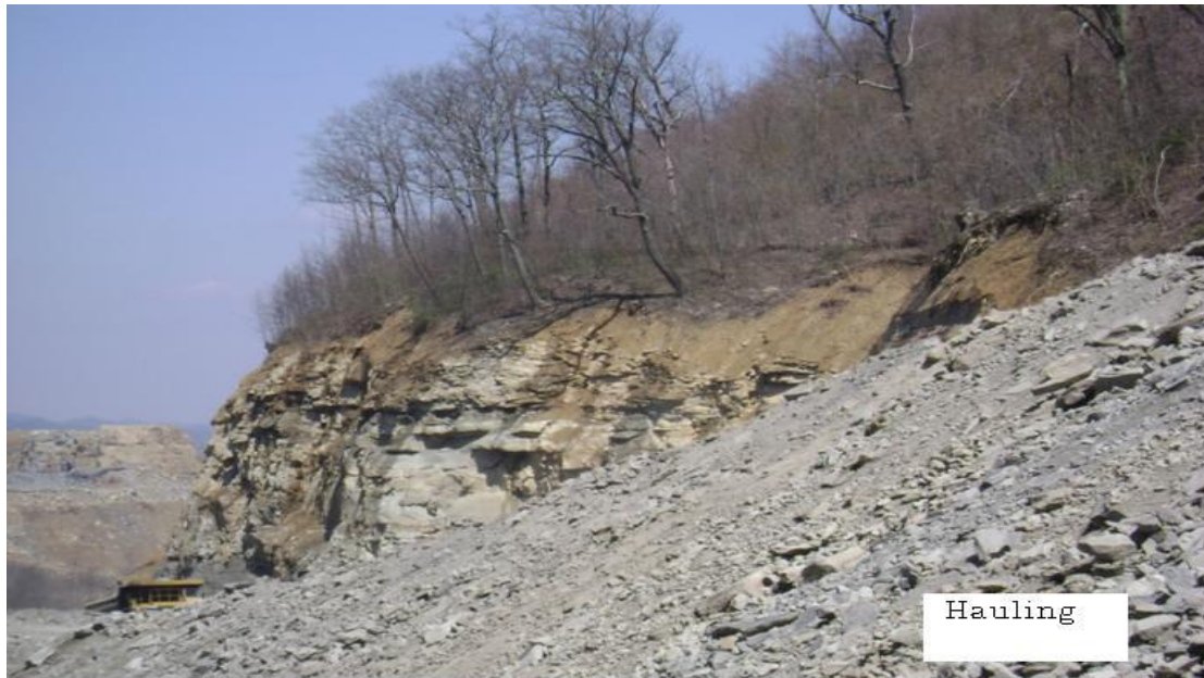
Figure 3: Hauling of spoil material
