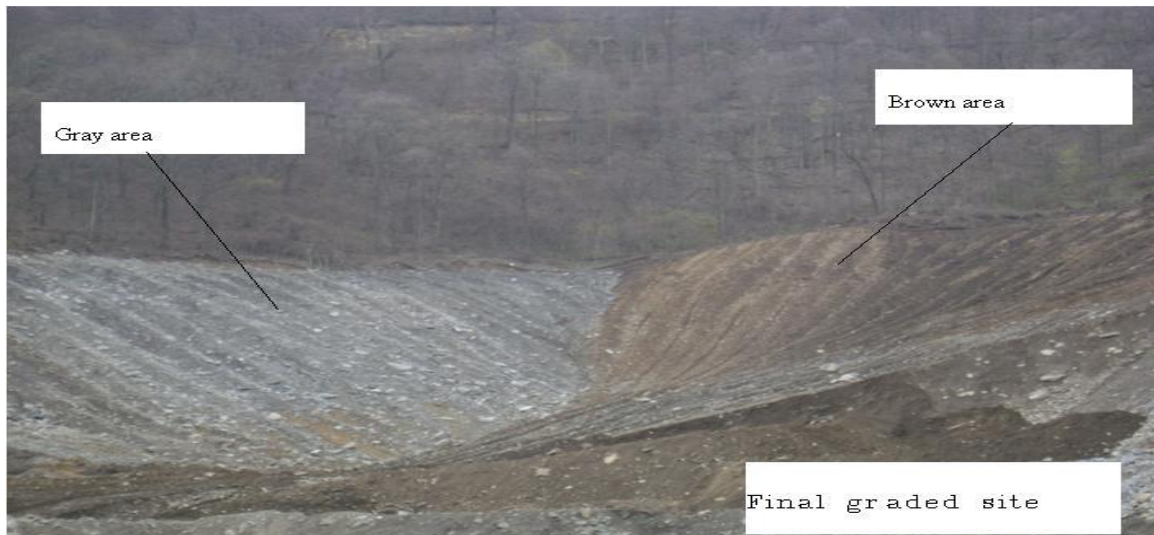
Figure 6: Site after final grading
