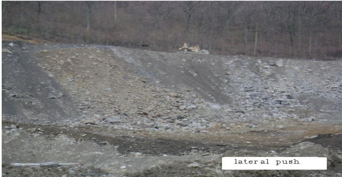
Figure 5: Lateral pushing of spoil material
