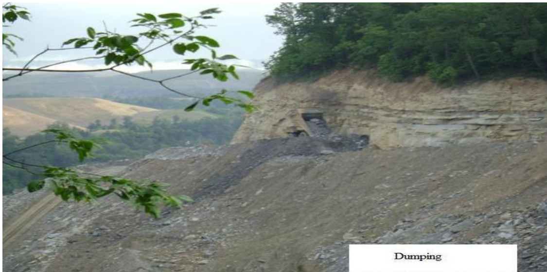
Figure 4: Dumping of spoil material
