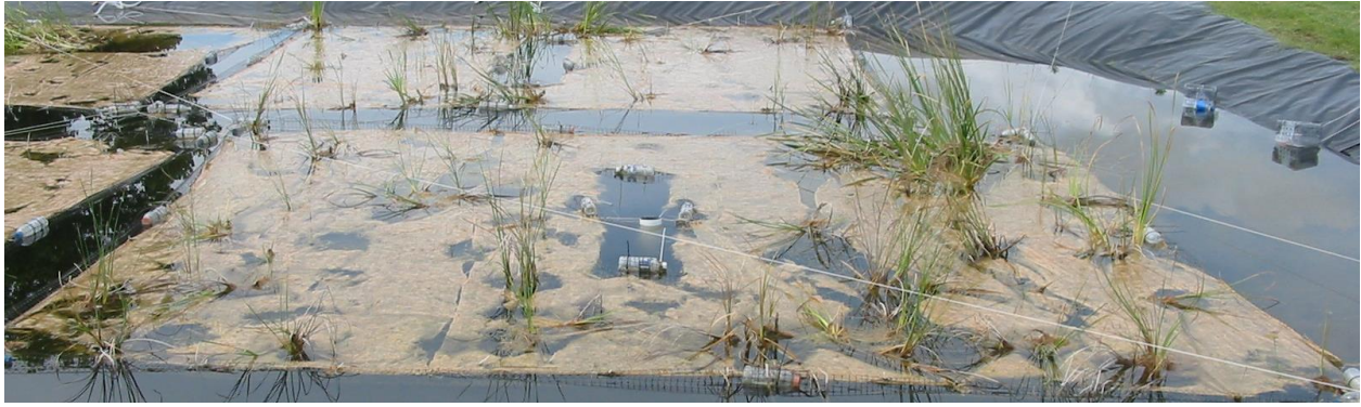
Figure 3. EFVM “E” approximately one year after construction and installation
