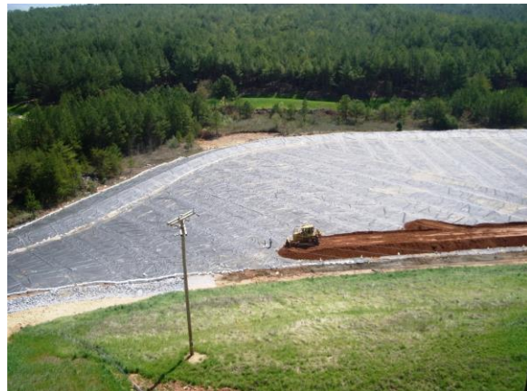
Figure 18. Tailings/Concentrate Area - During
