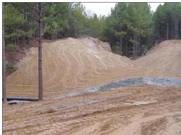
Figure 2. Tunnel Portal Area - After
