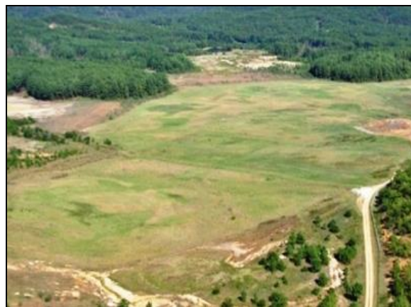
Figure 6. London Mill Tailings Pond 2007
