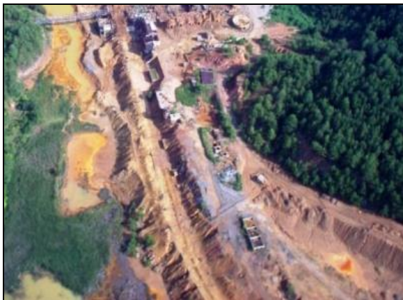
Figure 11. London Mill Shaft Area - Before
