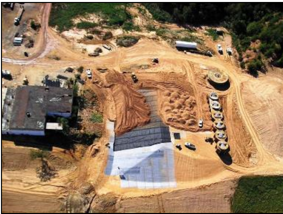
Figure 15. GCL at London Mill Flotation Plant
