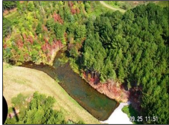
Figure 8. Low-Head Dam & Impoundment 2007
