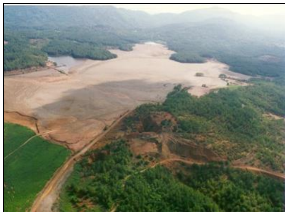
Figure 5. London Mill Tailings Pond 1993
