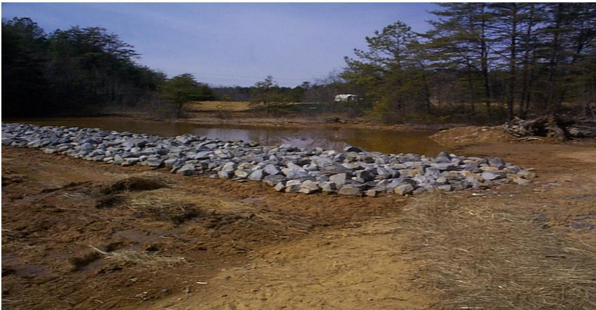
Figure 17. Berm 1 is in foreground forming Wetlands Cell 2; the new spillway over the dam shows in the background.
