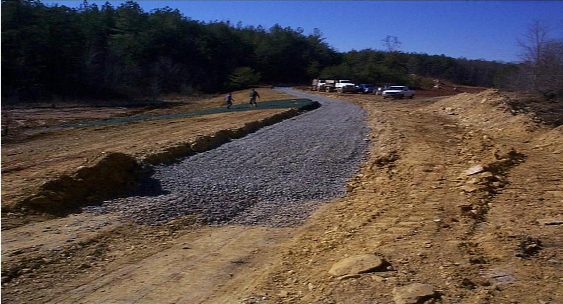
Figure 16. New 46 meter spillway cut into dam structure and reggraded dam face with vegetation mat on 5:1 slope.
