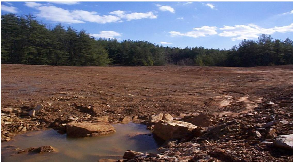
Figure 15. Soil cap over landfill containing wet-excavated spoils with microbial inhibitor applied.
