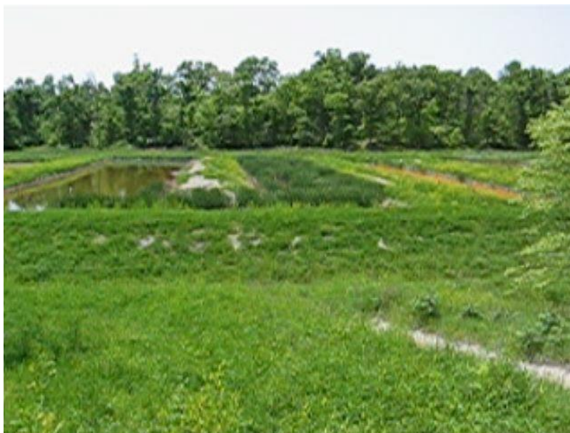
Figure 4. View of VFP #2 (left) and Aerobic Wetland #2 (center) - Photograph by OSM-MCRCC May 2003.
