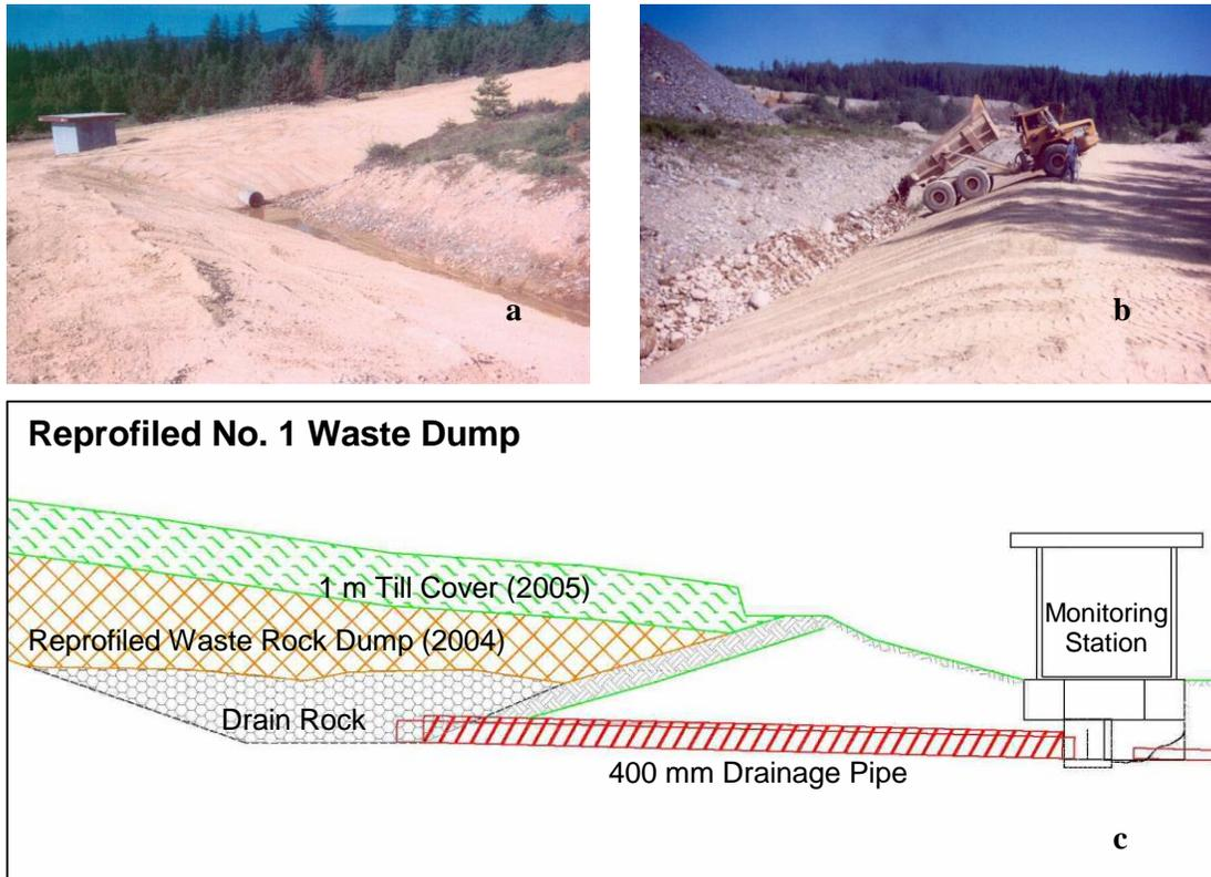
Figure 3. The monitoring station prior to reclamation (a). Drain rock being placed in the ditch (b). Cross-section showing drain rock, waste rock and till cover in former ditch with 400 mm pipe conveying seepage to monitoring station (c).
