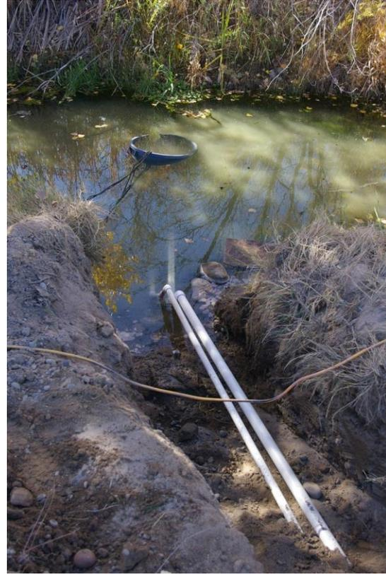
Photo 7. Influent pump container in the seepage trench with influent pipes.
