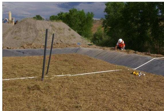
Photo 5. Substrate placement completed. Vertical standpipes are substrate sample ports.
