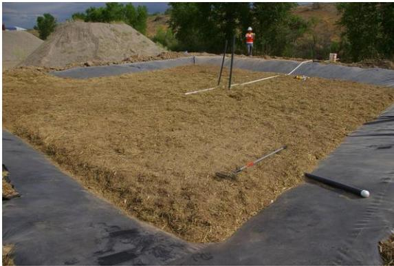
Photo 8. Influent pipe (white) extends to middle of cell. Drainage pipe cleanout in foreground (white end cap).
