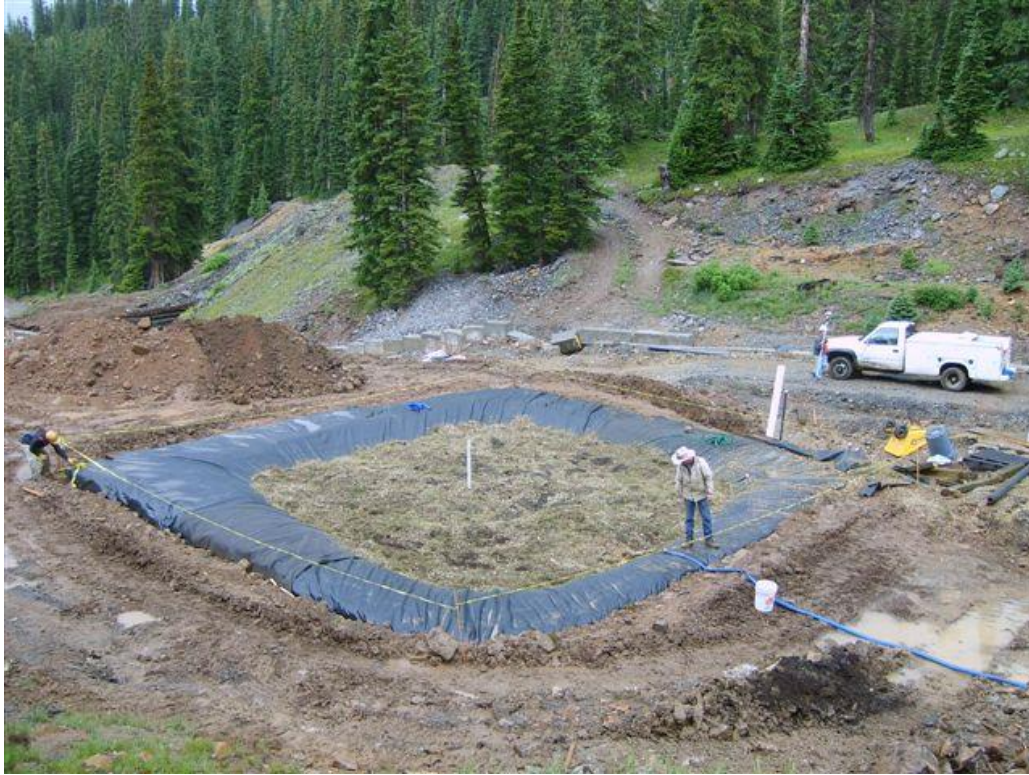
Figure 4 – Completed BCR Cell being filled with Incubation Water
