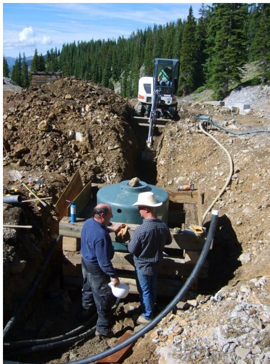
Figure 2 - Surge Tank Installation
