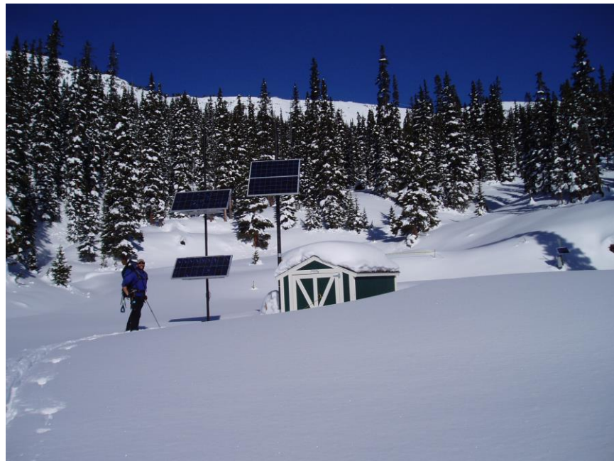
Figure 6 – Sample Shed and Solar Array
