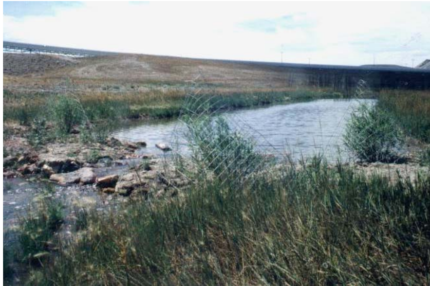
Figure 5: Pool and Counter-Weir Sequence on AVF Reach 1 with Caged Coyote Willow ( Salix exigua ) Plantings
