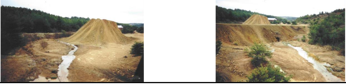
Figures 4. and 5. Refuse Pile near McPherson Branch caused water quality impact (see Table 1).
