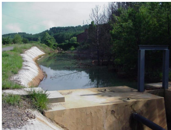
Figure 6. Concrete Diversion Dam.
